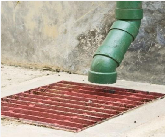
DRAINAGE WATER PIPE INSTALLATION
