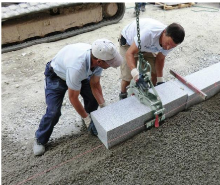
CONCRETE BLOCK INSTALLATION
